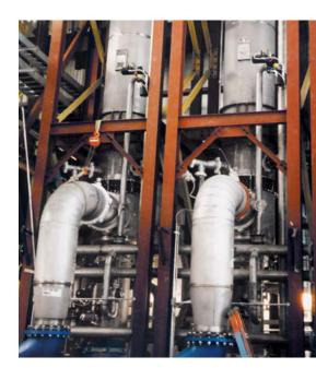
Vertically installed, multi-pass membrane modules in a multi-stage system design. Vertical configuration conserves floor space.
